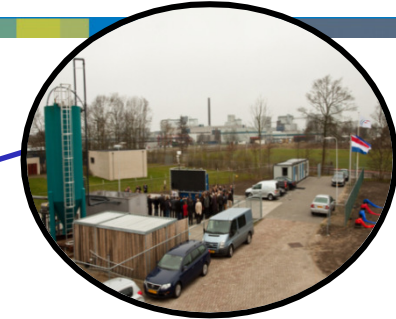
Municipal Waste Water Treatment
